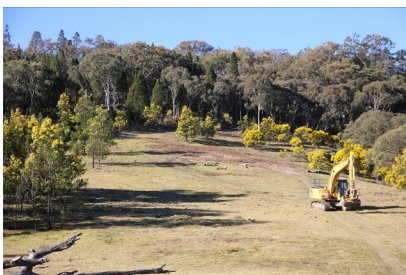
After final Environmental check, excavator leaves site.
