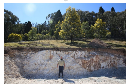
Tom from our Environment team showing scale of excavation.
