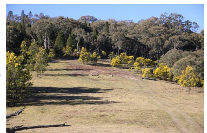
Earthworks complete and in this instance the site is left to naturally seed.
