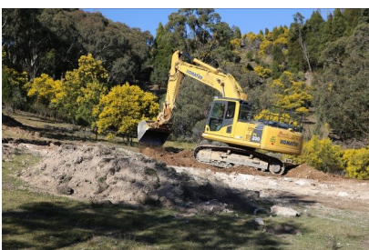
Topsoil layer is replaced on top of material and spread evenly across surface.
