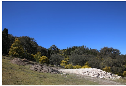
Side view showing extent of excavation. Note the separate topsoil piles.
