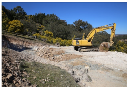
Earthworks contractor begins placing material back into original area.
