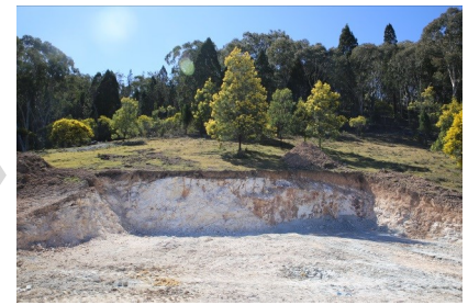
Front on view of excavated site demonstrating shallow topsoil layer.
